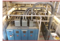
500 kW DC Power Supply 55 V / 9000 A 150 V / 3000 A
